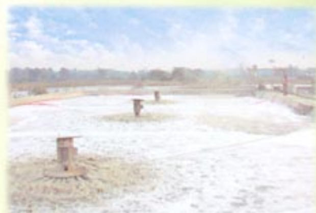
State-of-art Effluent Treatment Plant
